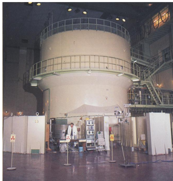
FIG. 1. RA reactor block.
