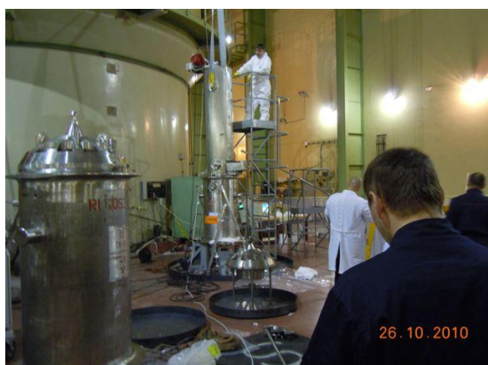
FIG. 14. Loading a basket into TUK-19 cask.
