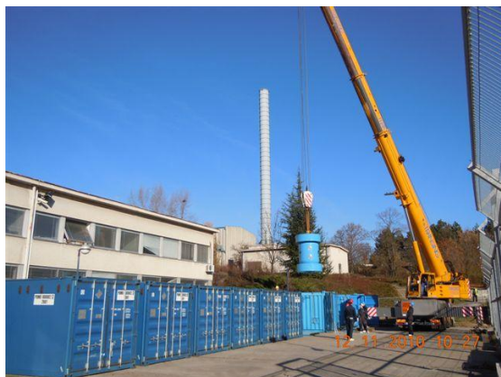
FIG. 17. Loading SKODA casks into ISO-containers.
